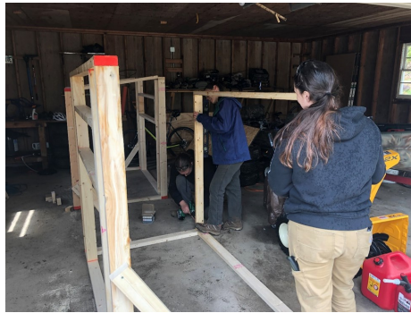
Caleb Hoernig, Hailey Hickok, and Lindsay Feather work on framing one of the two wildlife blinds.
